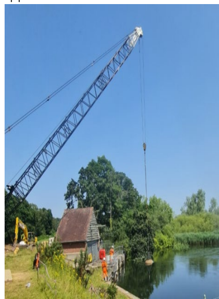
Matchams Intake - Riverbank Stabilisation
