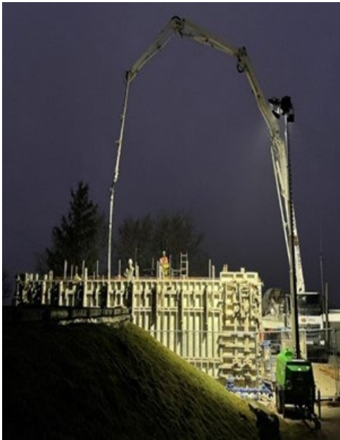
Hingston Down Service Reservoir under construction
